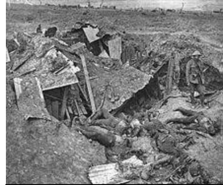
A demolished German trench and dugout near Guillemont
